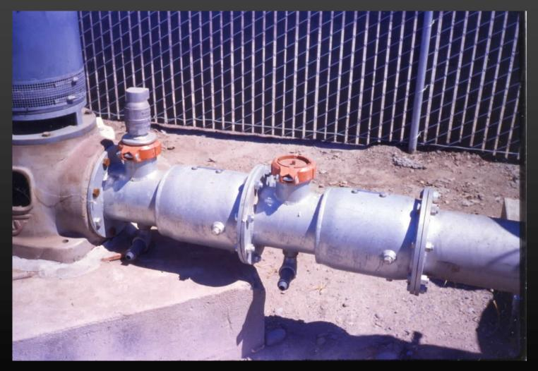
Some locales even require a *Pressure Reducing Backflow Prevention Valve*. These are the backflow prevention valves used on urban water systems and they are extremely expensive.
